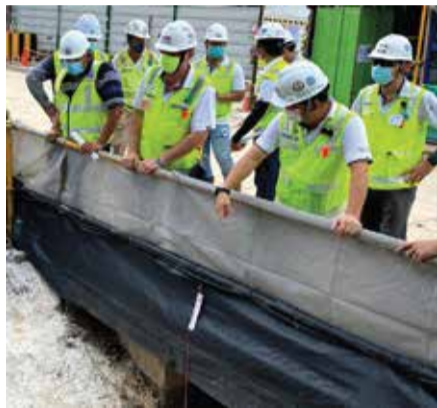
Top management EHS Site Inspection
